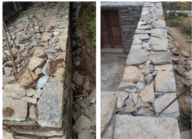
**Figure 2:** Multi leaf stone masonry construction in Ruby Valley, Dhading, Nepal (Photo taken: Sep-Dec 2018)
