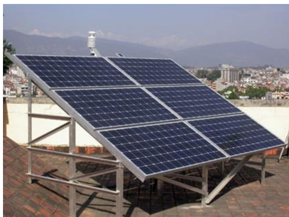
Figure 1: standard grid-connected 1.1 kWp PV plant at the CES (Centre of Energy Study) Pulchowk Engineering Campus of Tribhuvan University, Nepal's first Government University (P1)
