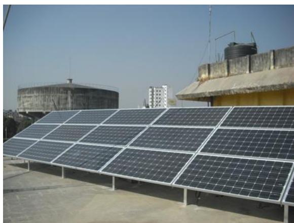
Figure 2: three 1.1 kWp PV systems were installed and connected to the grid at the NEA (Nepal Energy Authority) Min Bhawan office (P2)
