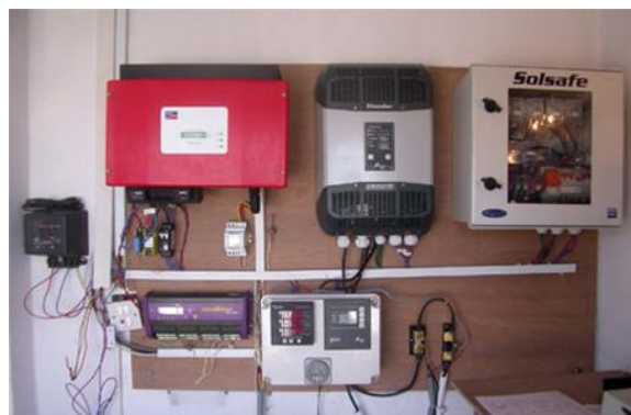
Figure 3: 1.1 kWp PV system with a back-up battery at the main head office of RIDS-Nepal in Imadol, Lalitpur district (P3)
