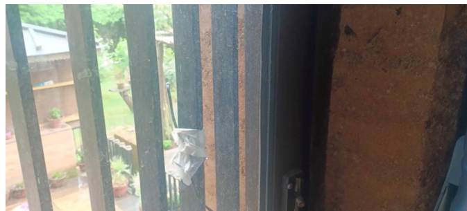
Figure 16: Measurement of Outdoor Temperature
