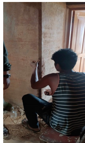
Figure 13: Applying Linseed oil finish at the walls
