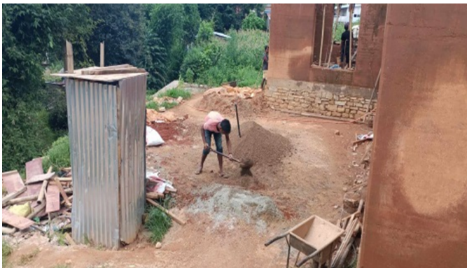
Figure 10: Mixing the rammed earth mixture manually
