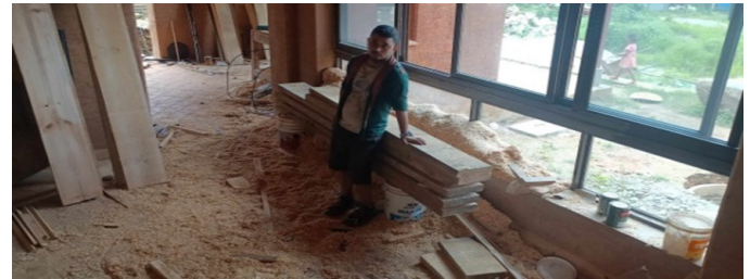
Figure 12: Wood works for flooring
