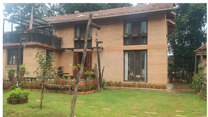
Figure 2: Reinforced Cement Stabilized Rammed Earth building at Godawari
