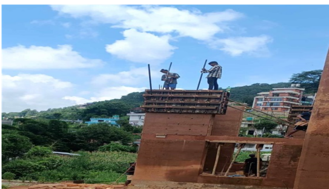
Figure 11: Ramming the Mixture
