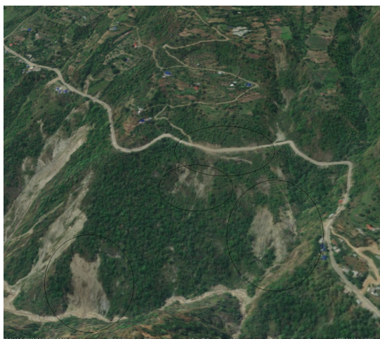
Figure 3: Settlement of road level and activation of local landslides at the bottom part of the slope
