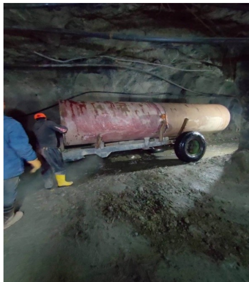
Figure 11: Transportation of penstock pipe to working station
