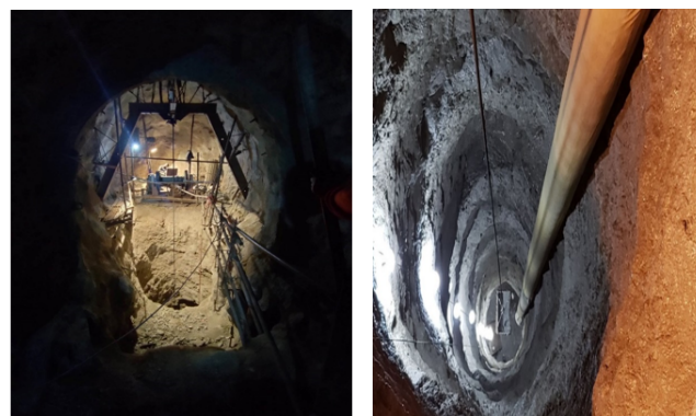
Figure 9: Hoisting platform (right) and Mucking out using Bucket (left)
