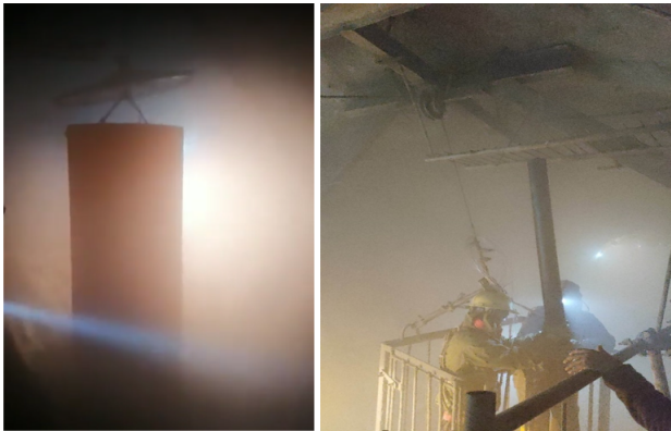
Figure 12: Post excavation activities: Lowering of penstock pipe (right) and Placing of PE pipe for backfilling (left)
