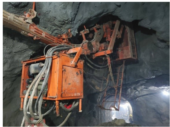
Figure 6: Vertical shaft excavation by using Rock climber method
