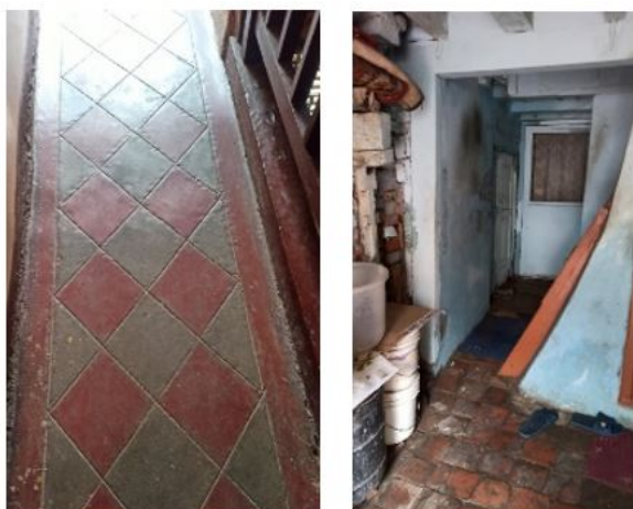
Figure 12: Use of Plaster and telia tiles in flooring
