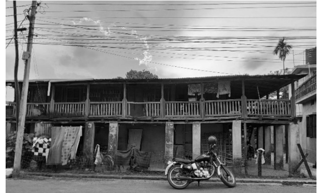
Figure 28: East elevation of the existing house
