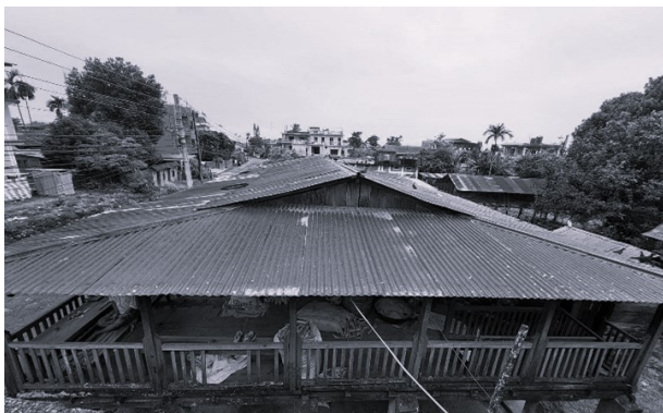
Figure 32: Northern balcony of the Main house
