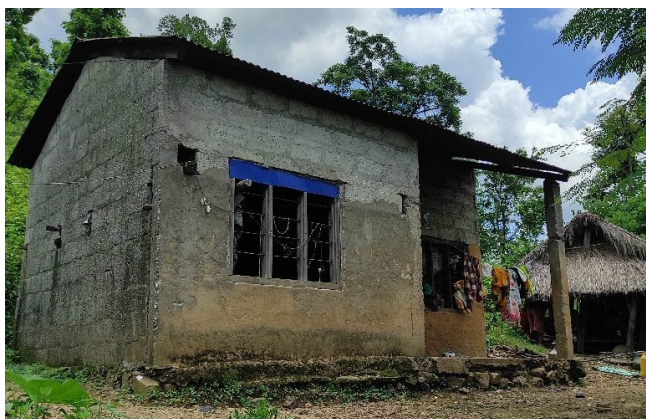
Figure 8: Cement Blocks in Walls
