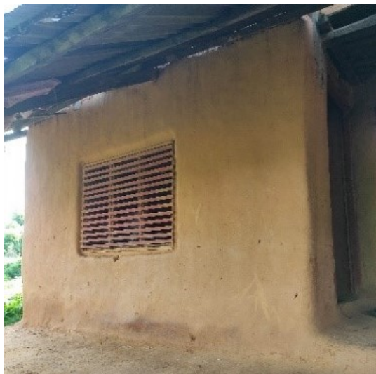
Figure 9: Stone Walls with Mud Mortar
