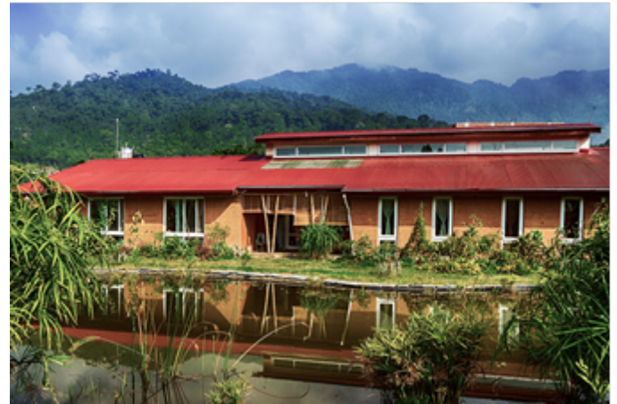
Figure 6.5: Matoghar, Budhanilkantha (Picture source: Prabal Thapa Architects)
