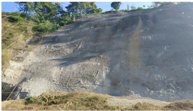
Figure 1: Soil nailing being done at Pasang Lambhu Highway at Dhading District
