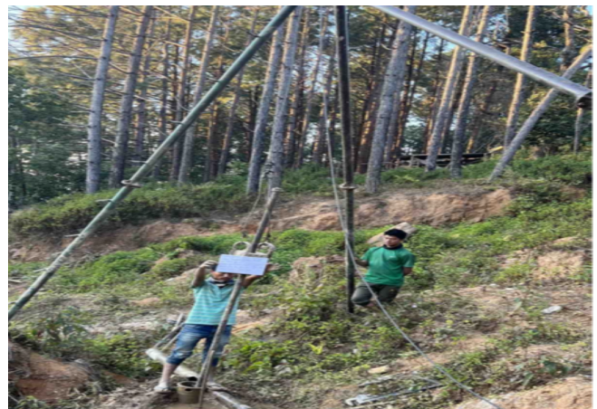
Figure 3: Site exploration being conducted at site
