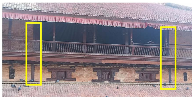
Figure 9: Use of wooden columns to strengthen the structure (Source: Author)
