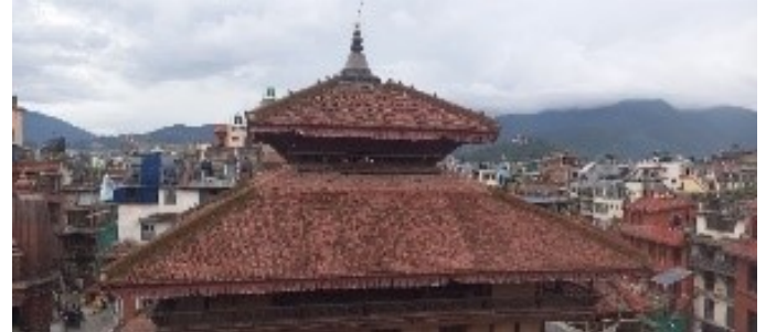
Figure 5: Metal gajur after reconstruction as in original design (Source: Author)
