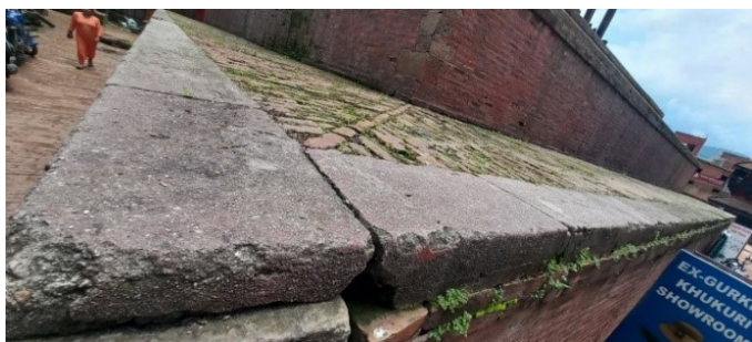
Figure 12: Replacement of stone with concrete (Source: Author)
