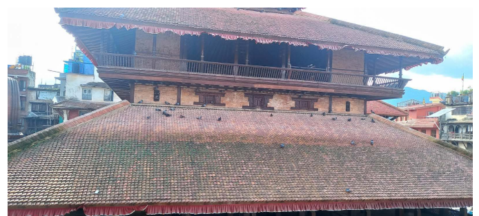
Figure 7: Raw brick wall exposed as original design (Source: Author)
