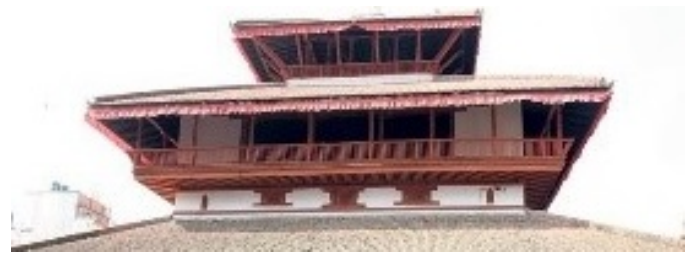
Figure 6: Use of lime wash before 2015 earthquake (Source: Author)
