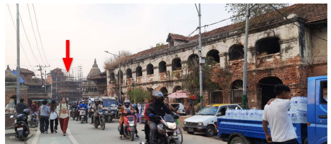
Figure 7: Bhaidega Temple after 2015 earthquake (Source: Author )
