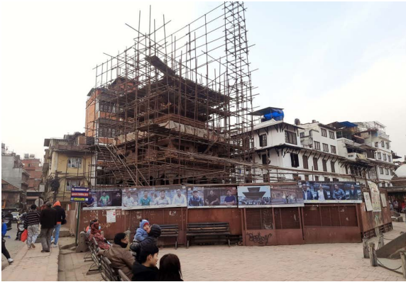
Figure 8: Bhaidega Temple after 2015 earthquake (Source: Author)
