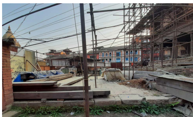
Figure 23: Dabali at eastern side of Bhaidega Temple Source: Author
