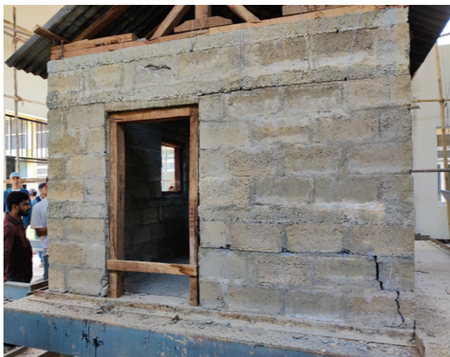
Figure 3: Failure pattern observed in the experimental model
