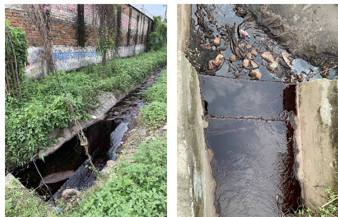
Figure 30: Waste water discharge from Dharan Industrial estate
