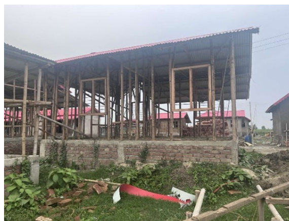
Figure 6: Bamboo frame structure used in houses
