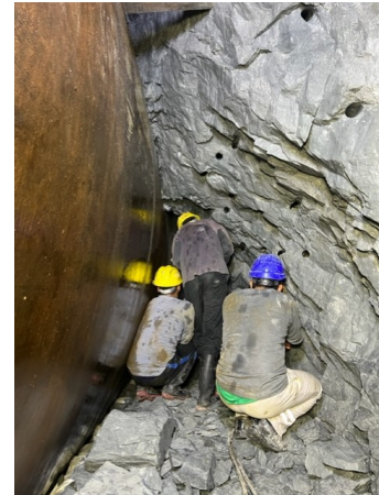
Figure 15: Bypass cavity excavation undergoing on right side at chainage 2+153m [5]
