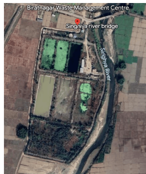
Figure 3: Aerial view of built up WWTP at BMC [6]
