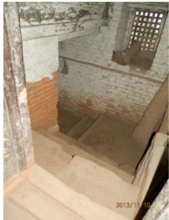
Figure 12: Mud plaster of staircase had crumbled down
