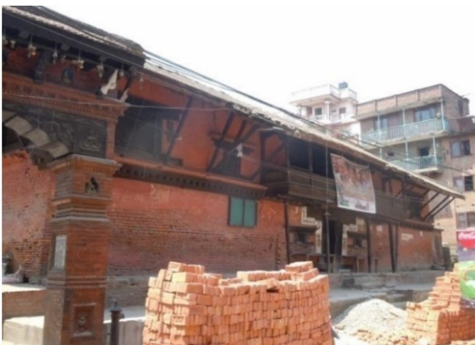
Figure 6: Dampness and Bulging out of Certain portions of the Outer Walls
