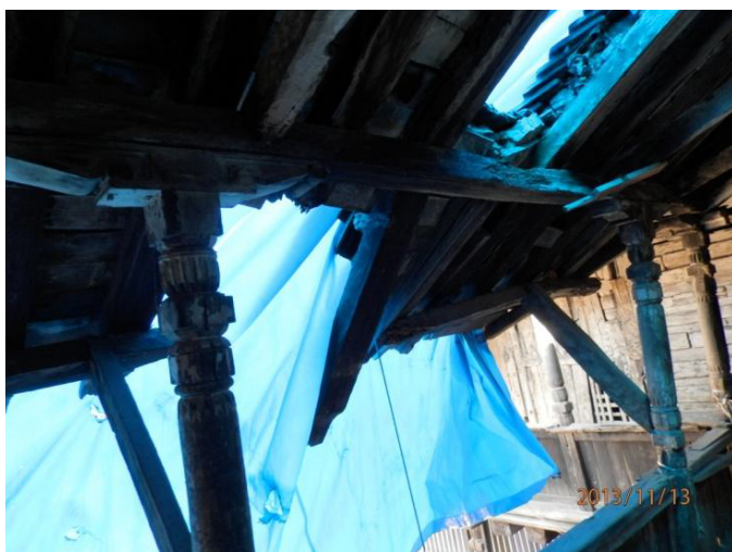
Figure 15: Hole on roof on the east wing. Presently this portion had conserved with the help of Department of Archeology
