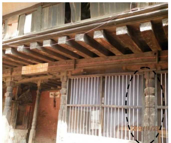
Figure 8: Tilted column and cracks on column
