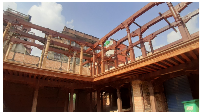
Figure 24: Use of old and new woodwork; shorter joists joined together to create longer joists
