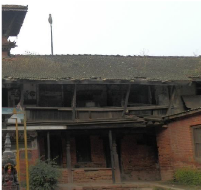
Figure 10: South Wing Verandah in bad condition
