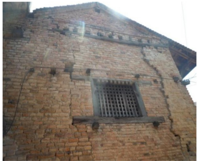
Figure 7: West Façade, Showing Cracks and Caving in of Walls
