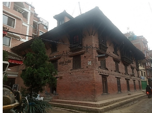
Figure 3: View of the Newa Chhen Building
