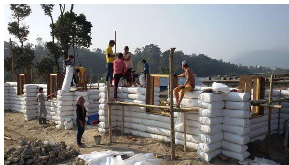
Figure 2: Earthbag Construction
