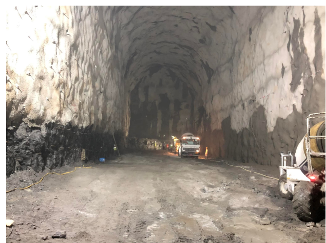
Figure 2: Powerhouse cavern of MMHPP
