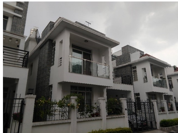
Figure 4: Houses at GHC, Lalitpur Source: author
