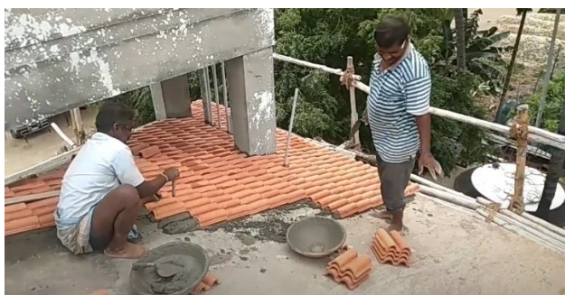
Figure 5: Locals laying khapra tiles over r.c.c building
