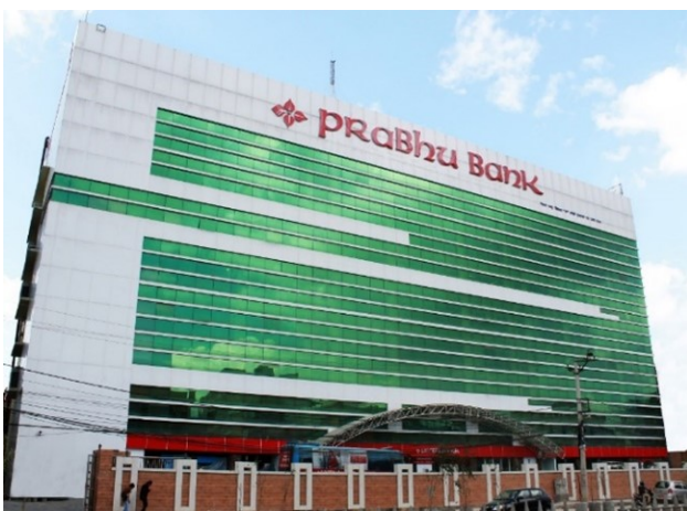
Figure 4: Front View of the Prabhu Bank (Prabhu Bank Limited)
