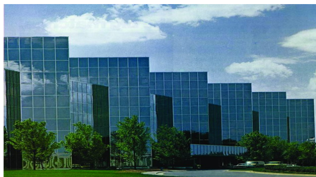
Figure 1: The use of new materials in building architecture[8]
