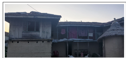
Figure 5: Typical traditional house in Kalaiya- Typology-5
