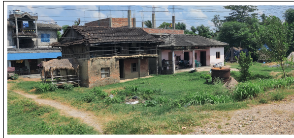
Figure 2: Typical traditional house in Kalaiya- Typology-2
