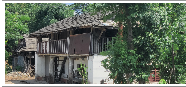
Figure 1: Typical traditional house in Kalaiya- Typology-1
