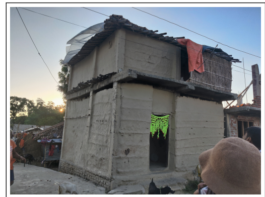
Figure 4: Typical traditional house in Kalaiya- Typology-4
