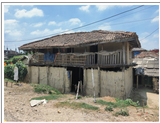
Figure 3: Typical traditional house in Kalaiya- Typology-3
