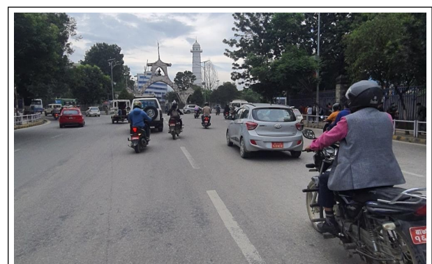
Figure 3: Good conditioned road
