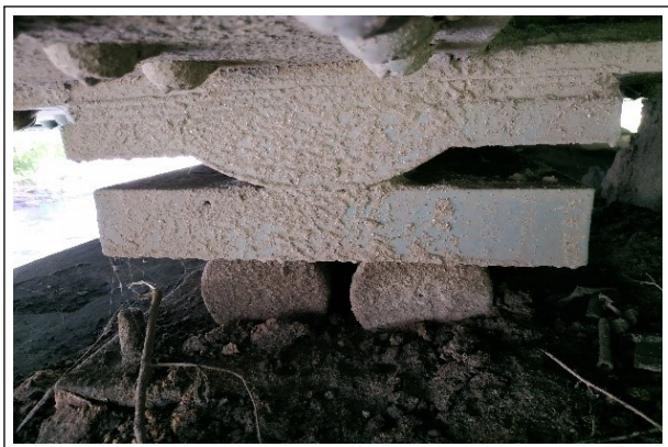
Figure 6: Roller Cum Rocker Bearing of the Bagmati Bridge
