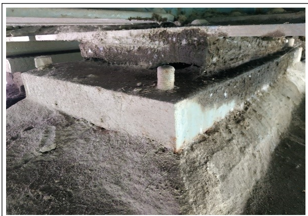
Figure 7: Rocker Bearing of the Bagmati Bridge
