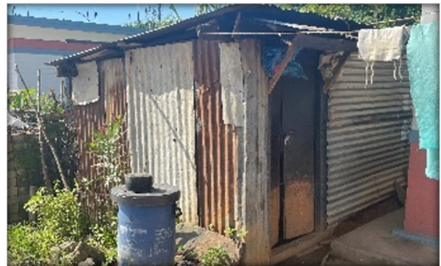
Figure 11: Temporary Shelter for Storage
