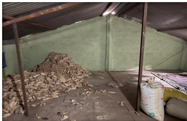
Figure 8: Attic used as Store
