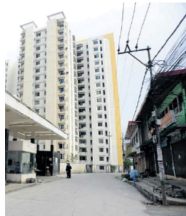
Figure 11: Façade treatment of the apartment
