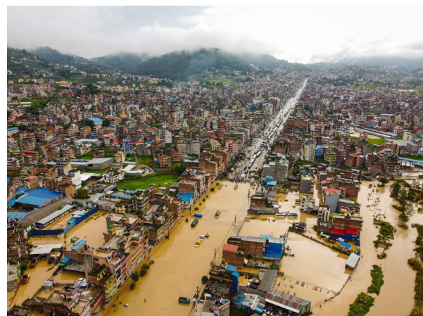
Figure 1: Urban Flooding in Banepa
