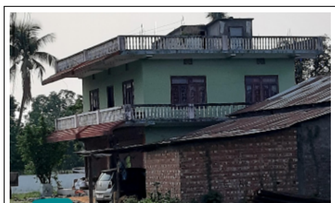
Figure 10: RCC: Modern Structures
