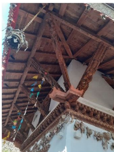
Figure 7: Carved cornice and struts in the south east corner
