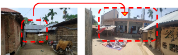
Figure 6: Replacement of mud house into RCC house; Residence of Mr. Ram Subaran Chaudhary after transformation
