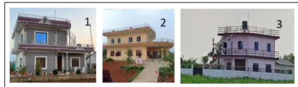
Figure 3: Modern residential building
