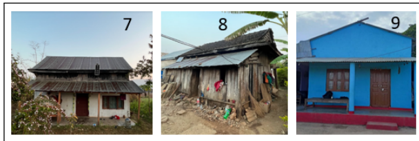
Figure 5: Hybrid residential building
