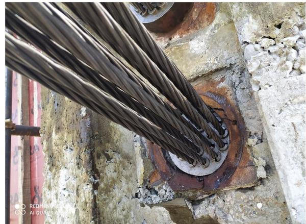
**Figure 21:** Anchorage failure during Post-tensioning
