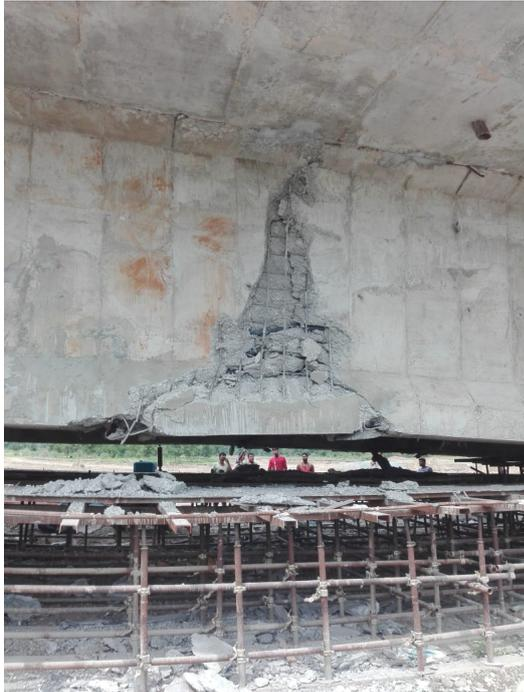
**Figure 22:** Beam failure during Post tensioning
