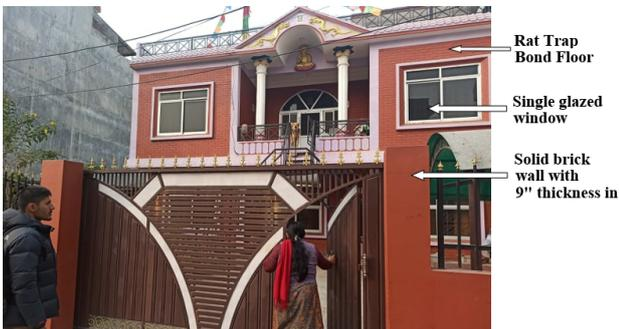
Figure 3: Building selected for simulation
