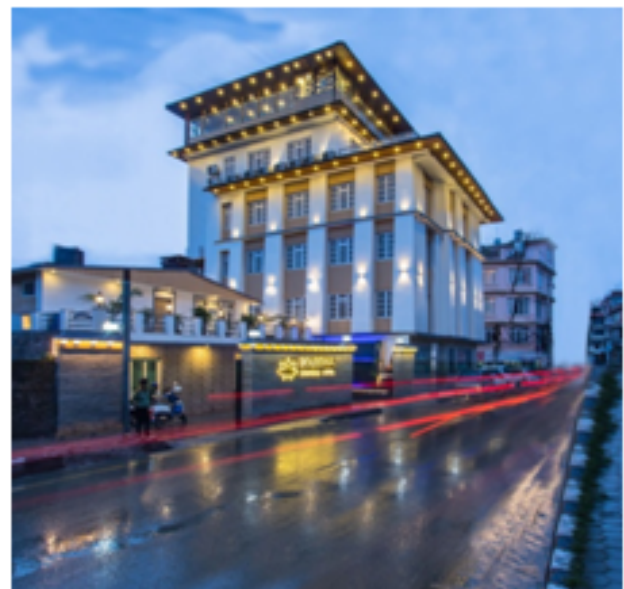
Figure 4: Existing Hotel Structure
