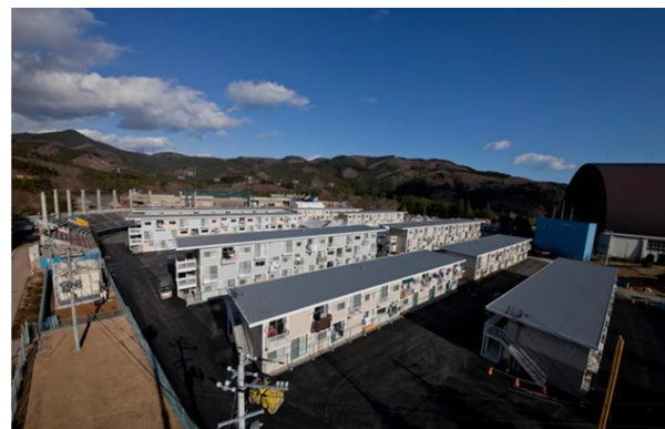
Figure 6: Onagawa Container, Miyagi, Japan
