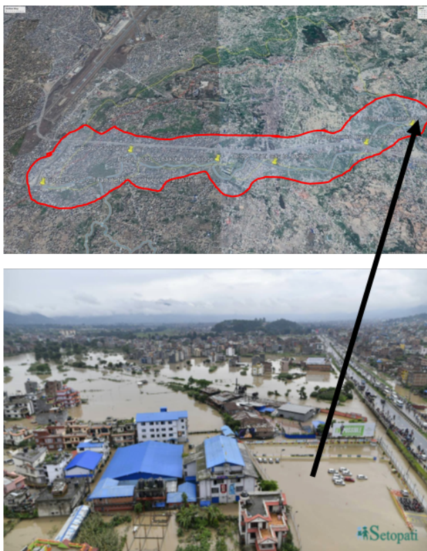
Figure 2: the affected area from flooding, settlements at Radhe Radhe and the Kamerotar land pooling project areas have become waterlogged on July 12th 2018 (Source: Setopati online news)
