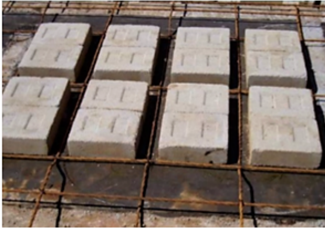
Figure 8: Filler Slab with CSEB as filler materials
