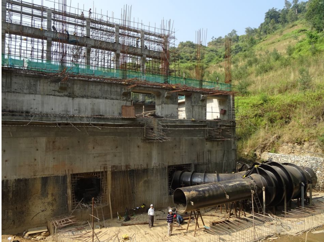
Figure 13: Bifurcation installed at site
