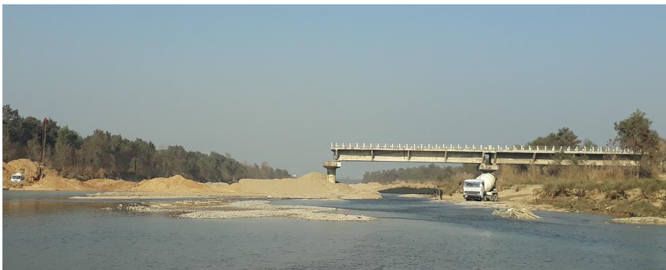
**Figure 1:** Tinau river bridge obstructed due to well sinking issues (Source: Bridge Branch, DoR, GoN)
