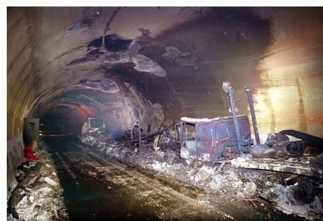
**Figure 1:** Damage caused by fire inside tunnel in Mont Blanc Tunnel [1]
