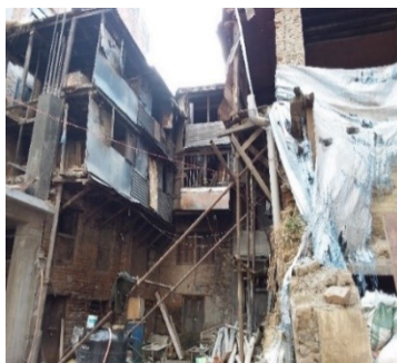
Figure 9: Vulnerable housing condition
