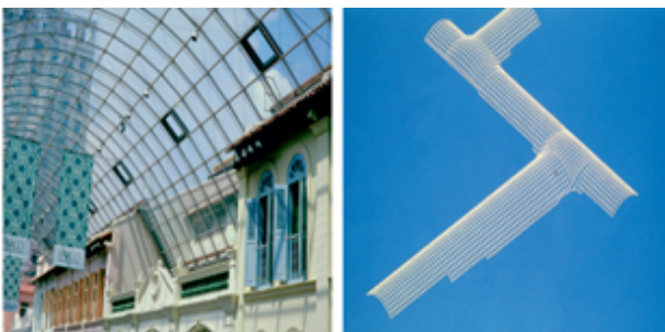
Figure 2: Roof Bugis Street Singapore [4]
